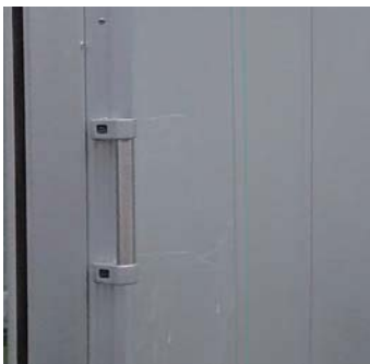
Aluminum opening/closing fitting with a handle for single leaf
